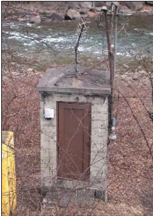
Figure 4. Example of a U.S. Geological Survey gaging station (USGS 01598500 NORTH BRANCH POTOMAC RIVER AT LUKE, MD)
